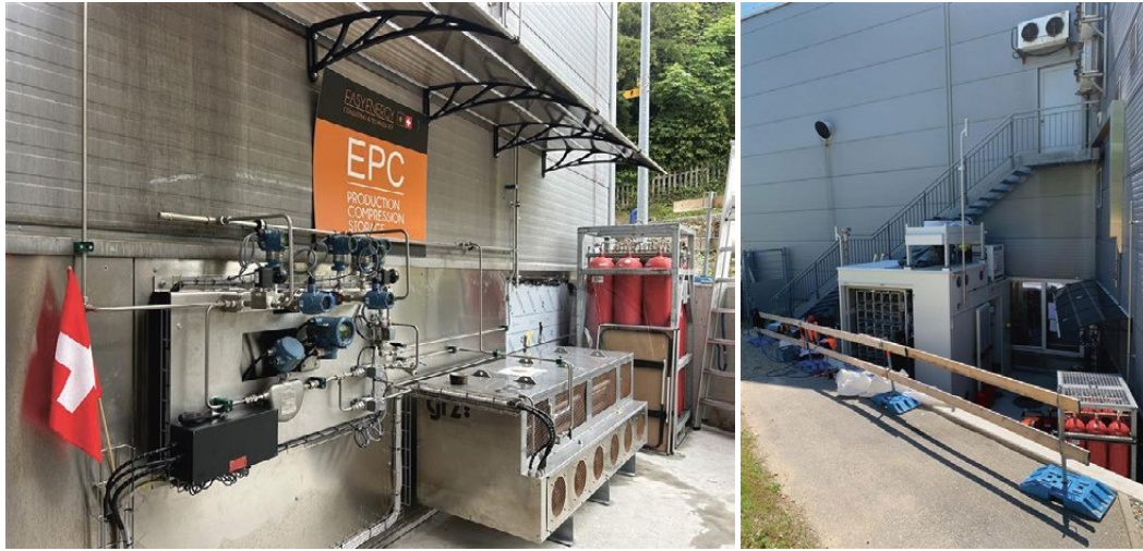
Figure 1 | Overview of EasyFlex installation on-site.
