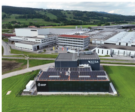
Figure 1 | Layout of the Gruyère Energie site with the Liebherr buildings just behind it.
